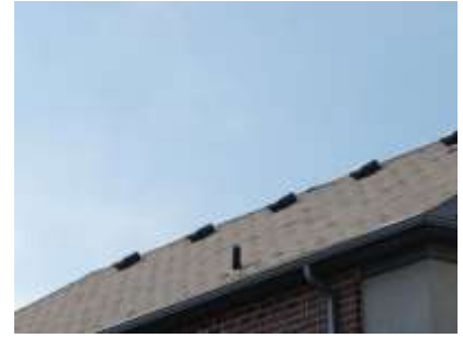
Pic. 3: Original roof covering
