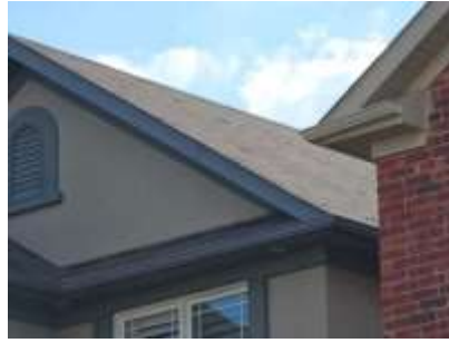
Pic. 2: Original roof covering
