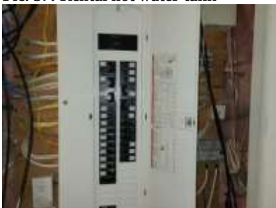
Pic. 40: 200 amp breaker panel
