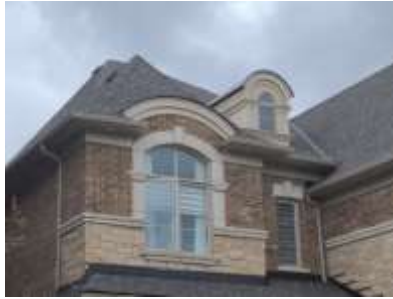
Pic. 2: Roof covering
