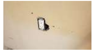
Pic. 8: Cover plates needed
