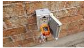
Pic. 3: Side outlet no power
