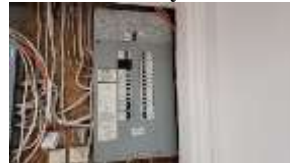
Pic. 43: 100 amp main electrical panel
