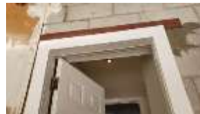
Pic. 11: Auto closer needed for garage entry door
