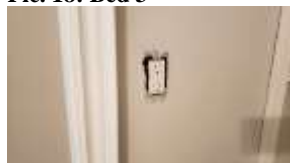
Pic. 22: Cover plate needed for outlet in bath
