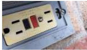
Pic. 6: Ground pin stuck in rear outlet
