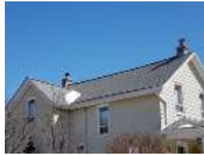
Pic. 2: Roof covering
