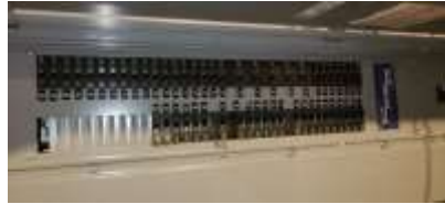
Pic. 47: 200 amp breaker panel
