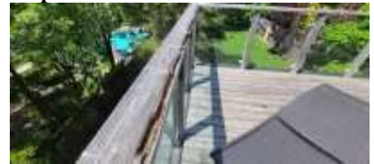
Pic. 12: Handrailing rot and should be replaced
