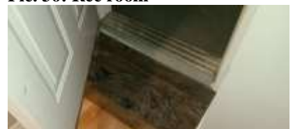
Pic. 39: Garage entry door opens onto steps – caution advised due to trip hazard
