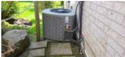
Pic. 10: AC unit 2012 – unit should be levelled
