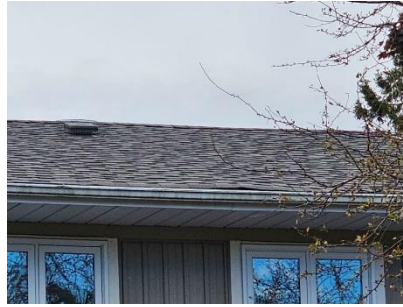
Pic. 2: Roof covering
