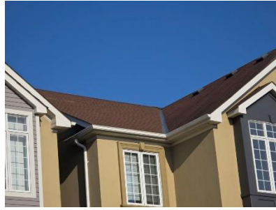
Pic. 2: Roof overhang
