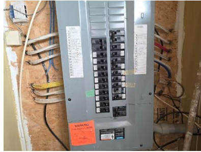
Pic. 32: 100 amp breaker panel
