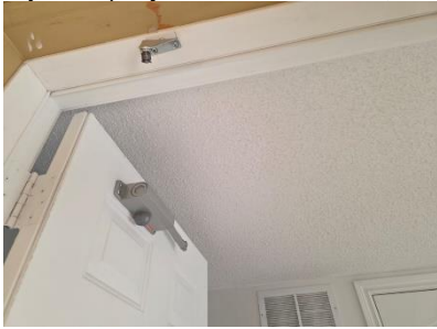
Pic. 31: Auto closer disconnected and damaged
