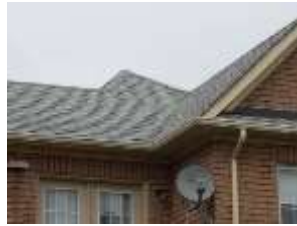
Pic. 2: Roof covering
