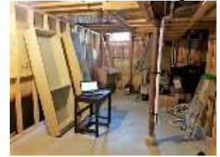
Pic. 24: Unfinished basement
