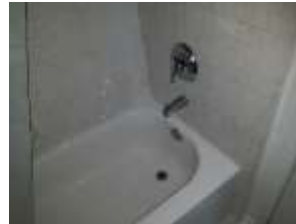
Pic. 15: 2 nd floor bath
