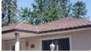
Pic. 2: Updated roof covering
