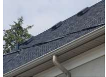
Pic. 3: Roof covering
