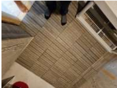
Pic. 26: Back flow preventor present
