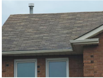
Pic. 2: Roof covering
