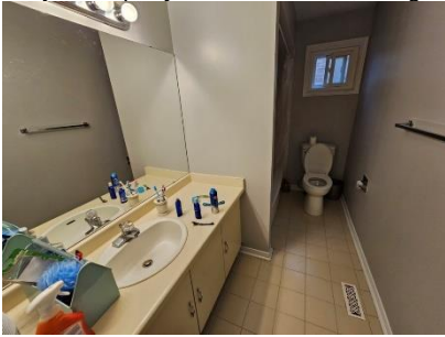
Pic. 16: 2 nd floor bath
