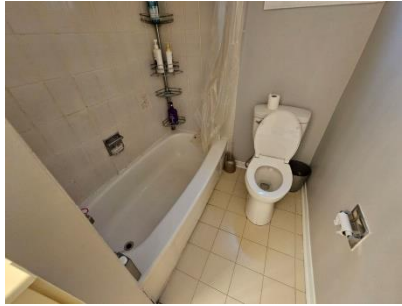
Pic. 17: 2 nd floor bath
