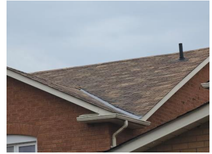
Pic. 3: Roof covering
