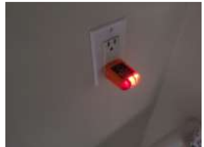
Pic. 30: GFCI outlet in powder room should be replaced
