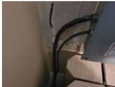
Pic. 38: Wiring needs to be properly secured
