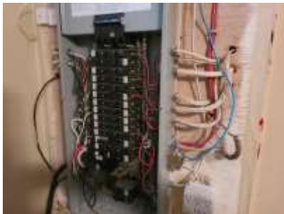
Pic. 37: 200 amp breaker panel
