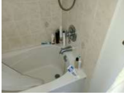
Pic. 20: 2 nd floor bath
