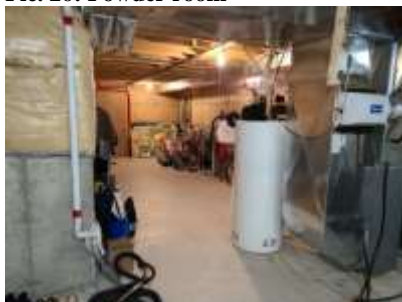
Pic. 29: Unfinished basement
