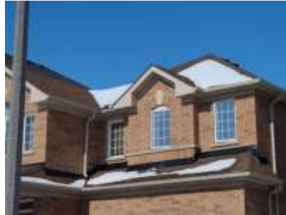
Pic. 2: Original roof covering
