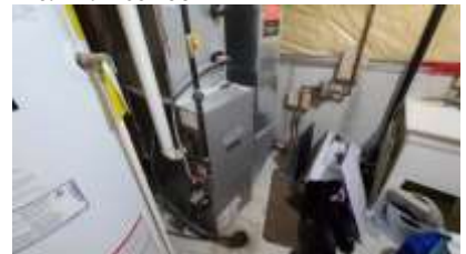
Pic. 27: Original gas furnace
