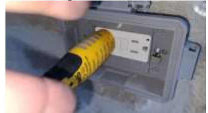
Pic. 6: Front GFCI has no power
