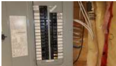
Pic. 29: 100 amp breaker panel
