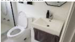
Pic. 21: Basement bath
