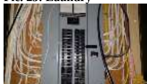
Pic. 27: 100 amp breaker panel with all copper wire
