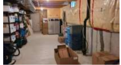
Pic. 24: Unfinished basement
