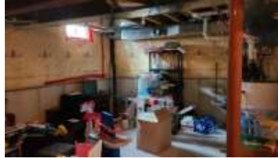
Pic. 23: Unfinished basement
