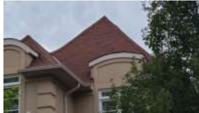
Pic. 2: Original roof covering
