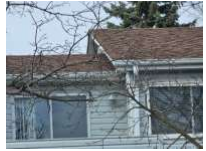
Pic. 3: Updated roof covering
