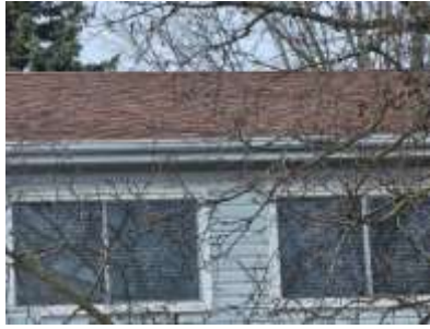
Pic. 2: Updated roof covering
