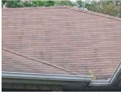
Pic. 2: Roof covering
