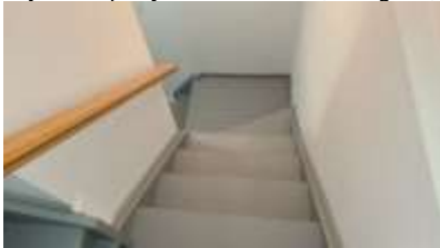
Pic. 19: Basement stairwell – stairs have an uneven rise
