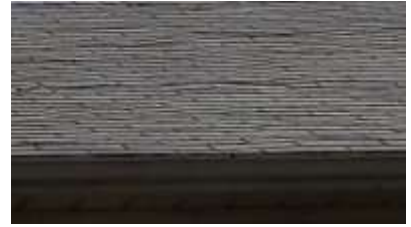
Pic. 3: Signs of warping of the roof sheathing due to lack of ventilation in the attic
