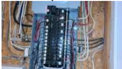
Pic. 26: 100 amp breaker panel
