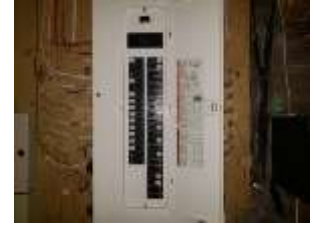
Pic. 32: 200 amp breaker panel
