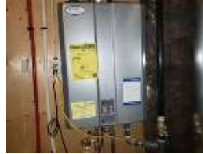
Pic. 31: Tankless hot water
