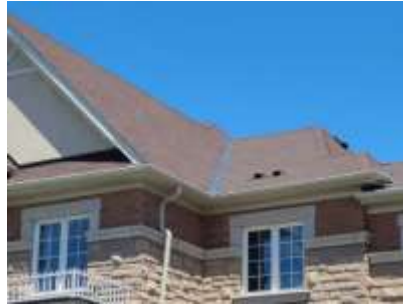
Pic. 2: Roof covering
