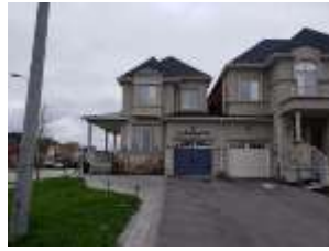
Pic. 2: Garage view
