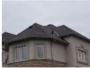
Pic. 2: Roof covering
