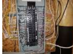
Pic. 43: All copper wire
