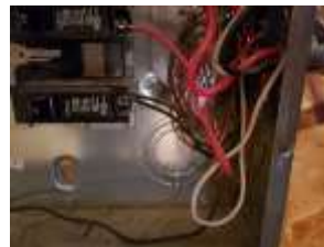
Pic. 35: Double tapped breaker
