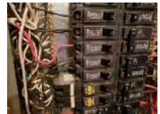
Pic. 36: Double tapped breaker
