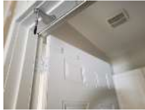
Pic. 6: Working auto closer required for entry door to garage
