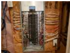
Pic. 34: 150 amp breaker panel
