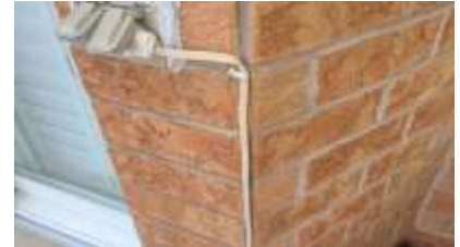
Pic. 6: Handyman extension cord wiring in backyard should be reviewed and corrected accordingly
