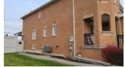
Pic. 3: Side view
