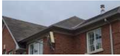
Pic. 2: Roof covering
