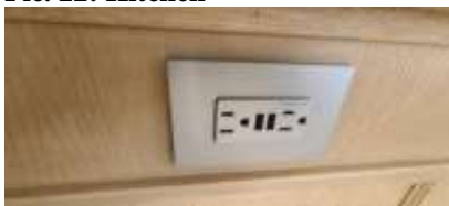
Pic. 25: Island outlet should be GFCI protected
