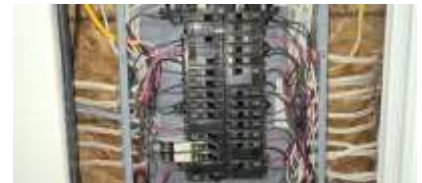
Pic. 35: 100-amp breaker panel
