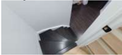
Pic. 28: A handrailing is needed for the basement stairwell
