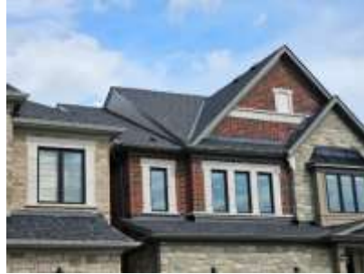
Pic. 2: Roof covering
