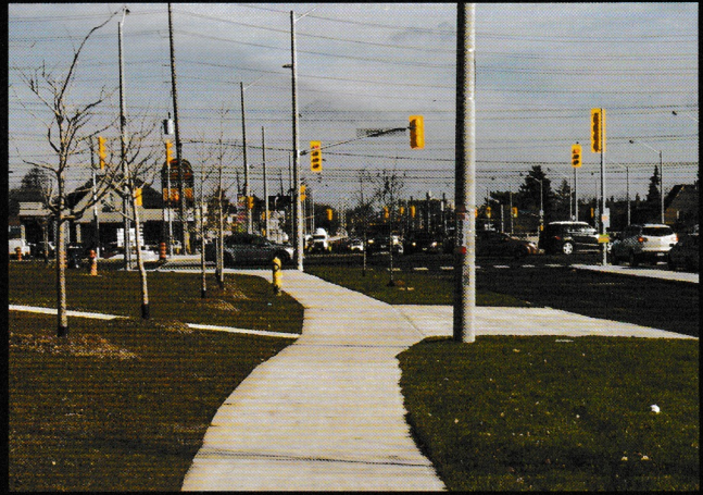
Photo: Permanent traffic signals at Finch Avenue West and Highway 27 intersection, view east.
