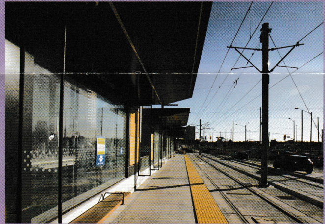
Photo: Jane and Finch platform, rails and overhead catenary system.
