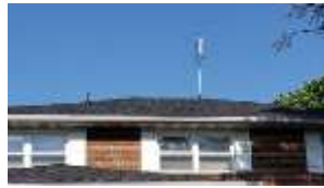
Pic. 2: Updated roof covering
