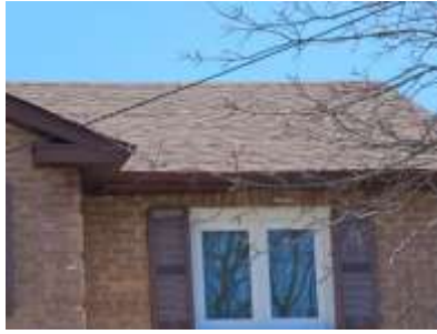
Pic. 2: Updated roof covering
