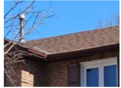
Pic. 3: Updated roof covering
