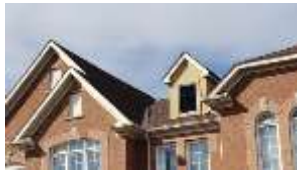
Pic. 2: Updated roof covering
