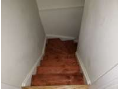
Pic. 18: Handrailing needed in basement stairwell
