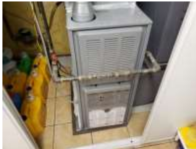
Pic. 22: Mid efficiency gas furnace
