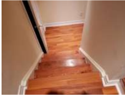
Pic. 19: Handrailing needed in basement stairwell
