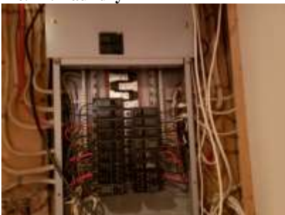
Pic. 24: 100 amp breaker panel with all copper wire
