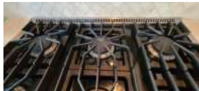
Pic. 29: Rear middle burner not operating – control knob broken
