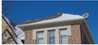
Pic. 2: Visible roof covering
