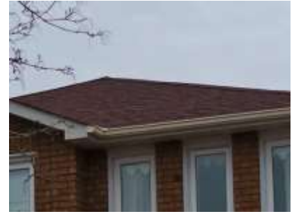
Pic. 3: Updated roof covering
