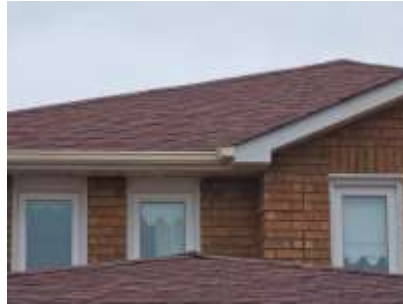
Pic. 2: Updated roof covering
