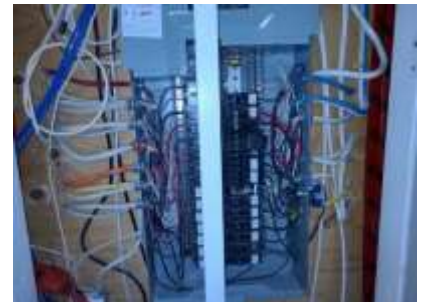
Pic. 27: 100 amp breaker panel
