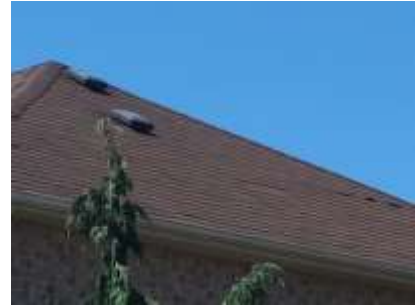
Pic. 3: 1 missing shingle tab and some cupping of the roof covering
