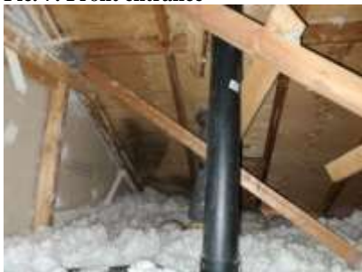
Pic. 10: Attic – one section with old staining – no active moisture present
