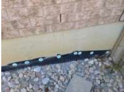
Pic. 4: Typical foundation settlement crack
