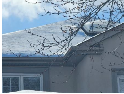
Pic. 2: Roof covering snow covered
