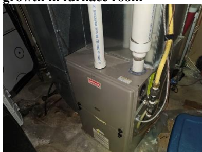
Pic. 41: Gas furnace 2012
