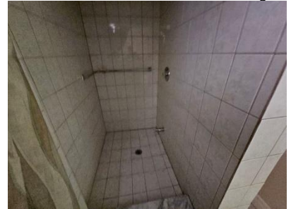
Pic. 33: Basement bathroom
