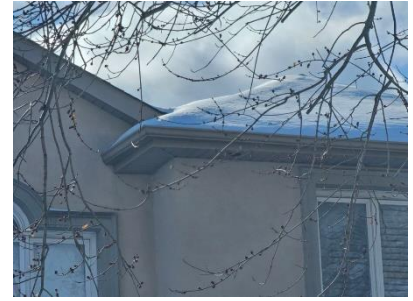
Pic. 3: Roof covering snow covered
