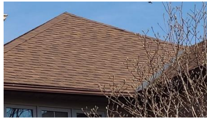
Pic. 2: Updated roof covering
