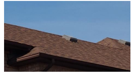
Pic. 3: UYupdated roof covering
