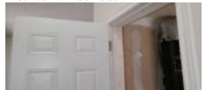
Pic. 18: Auto closer required for garage entry door
