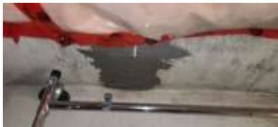
Pic. 28: Professionally repaired foundation crack
