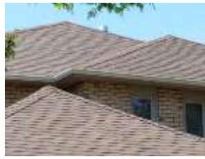
Pic. 2: Roof covering
