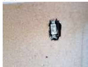
Pic. 11: Switch cover missing
