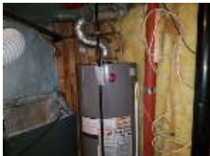
Pic. 41: Rental hot water tank
