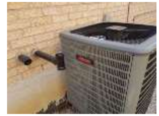
Pic. 4: AC Unit
