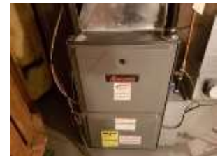
Pic. 40: High efficiency gas furnace
