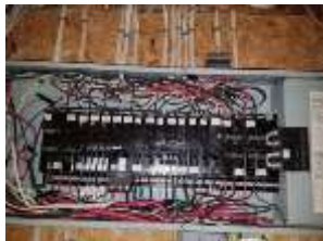
Pic. 42: 200 amp breaker panel with all copper wire. One breaker double tapped and two breakers oversized
