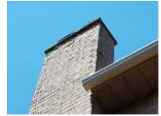
Pic. 8: Chimney with some flaking of bricks
