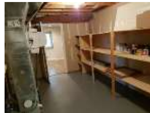
Pic. 39: Utility room
