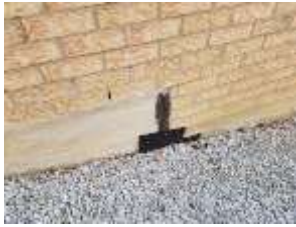
Pic. 5: Repaired foundation crack
