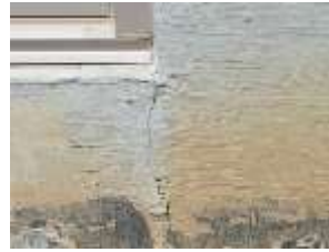
Pic. 7: Typical foundation crack
