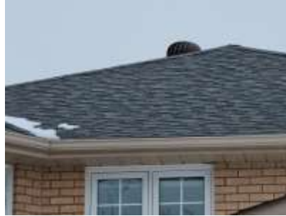
Pic. 2: Updated roof covering
