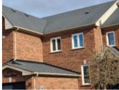
Pic. 2: Updated roof covering
