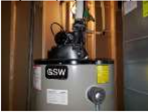
Pic. 41: Rental hot water tank
