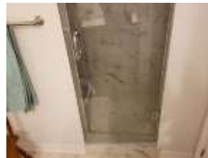
Pic. 39: Basement bath
