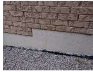
Pic. 3: Typical foundation crack – so indications of water seepage issues
