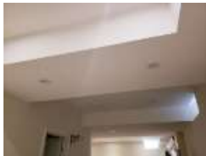
Pic. 34: Pot light three way switched wired incorrectly
