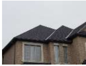
Pic. 2: Roof covering
