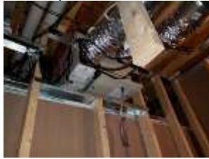
Pic. 42: HRVC poorly located for service and cleaning
