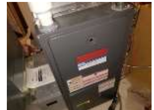
Pic. 40: High efficiency gas furnace
