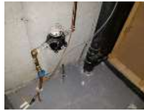
Pic. 39: Water main panel
