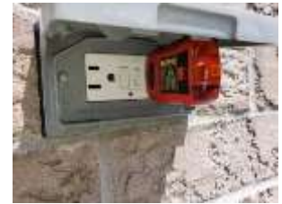
Pic. 4: Rear GFCI needs replacement
