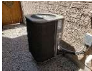
Pic. 2: AC unit 2008
