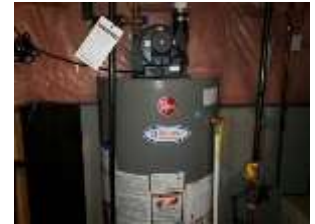
Pic. 36: Rental hot water tank
