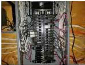
Pic. 38: 200 amp breaker panel
