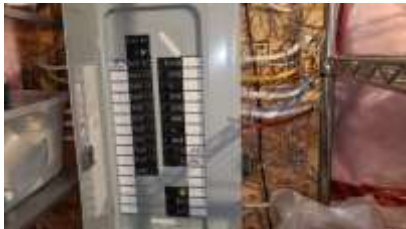
Pic. 13: 100 amp breaker panel
