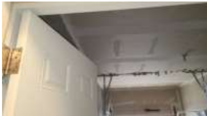
Pic. 7: No auto closer on garage entry door
