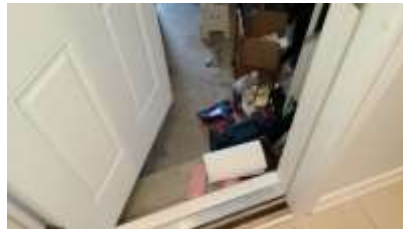
Pic. 8: Garage entry door opens into the garage step – trip hazard
