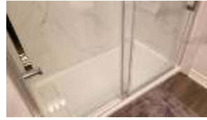
Pic. 35: Basement bath
