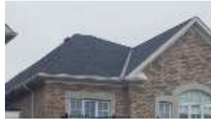
Pic. 2: Roof covering
