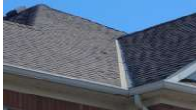
Pic. 2: Updated roof covering
