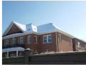
Pic. 2: Roof covering snow covered
