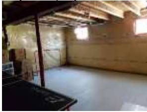
Pic. 25: Unfinished basement
