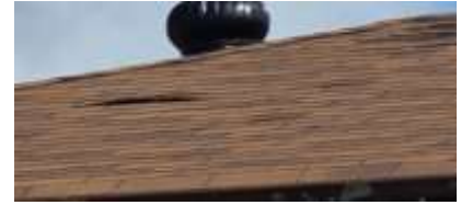
Pic. 3: Review and some repairs required
