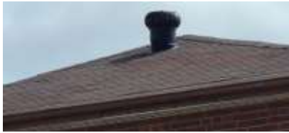
Pic. 4: Review and some repairs required
