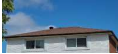
Pic. 2: Roof covering
