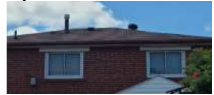
Pic. 6: Rear roof covering
