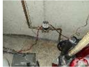
Pic. 27: Water main
